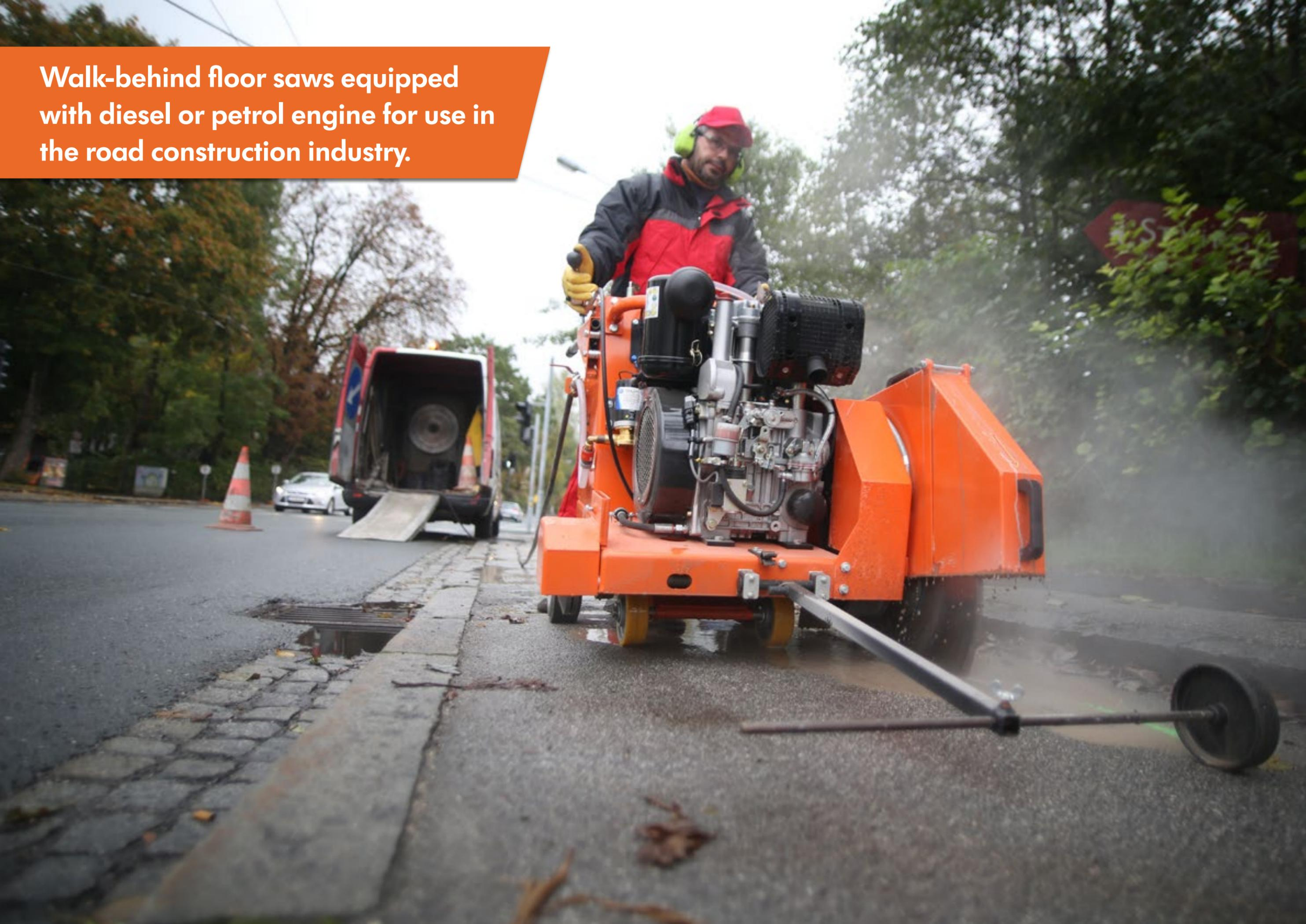
**Self propelled Concrete and Asphalt Saw - electrically driven - The powerful and compact solution for medium-large sawing jobs in asphalt and concrete roadworks**
